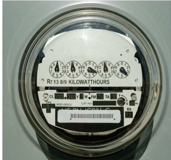
Household Electrical Meter
