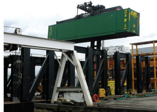
Container is unloaded from shipping barge
