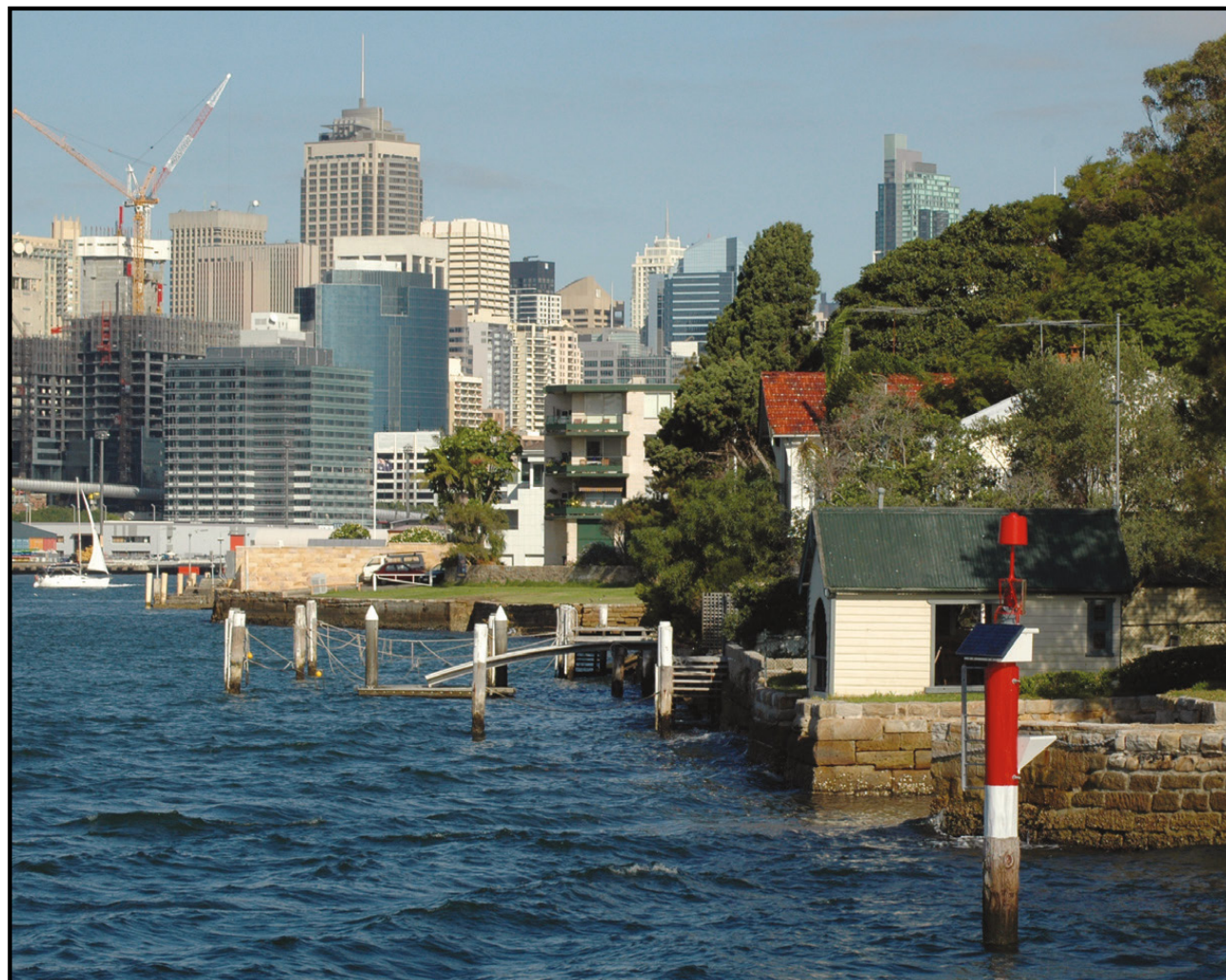
Sea retaining wall — Sydney, AU
